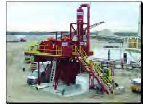
PHOTO #4 - Sand Plant
